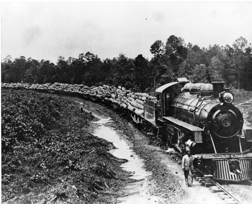
Photo 6: Train transporting flat cars of logs in Ashley County, not dated (Ashley County Scenes Photograph Collection, ca. 1900-1979)
