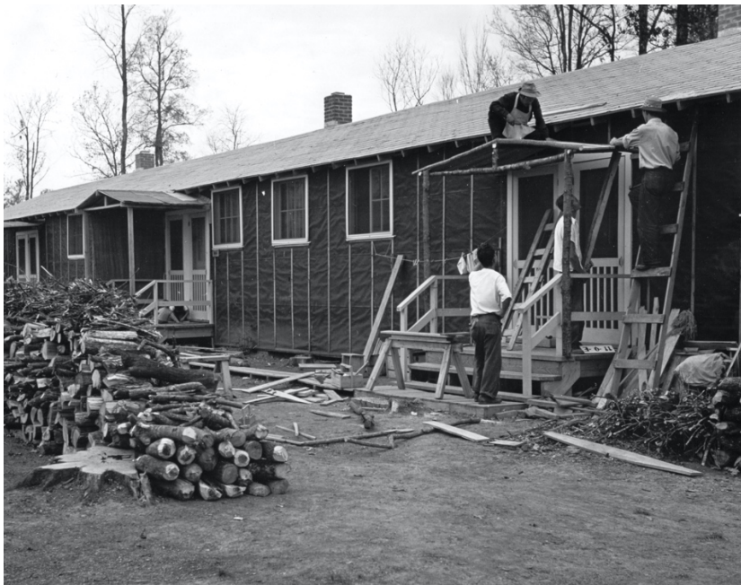
Photo 2: Three men build a porch cover for a barracks doorway at Rohwer Relocation Center, ca. 1942-45 (Life Interrupted Collection, 1903-2005)
